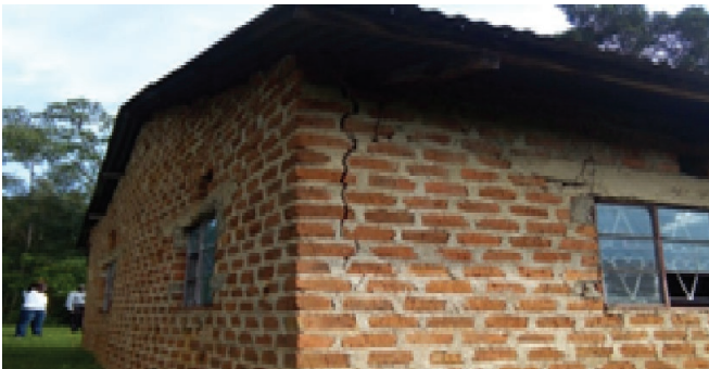
Cracked wall for house near the quarry (By Benson Khamasi)
