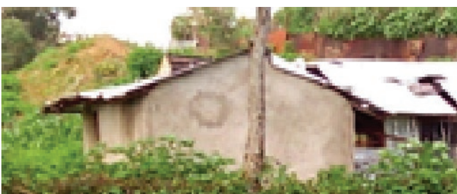
House roof damaged by flying rock (By Benson Khamasi)
